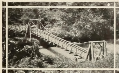
Thunder Creek suspension bridge
